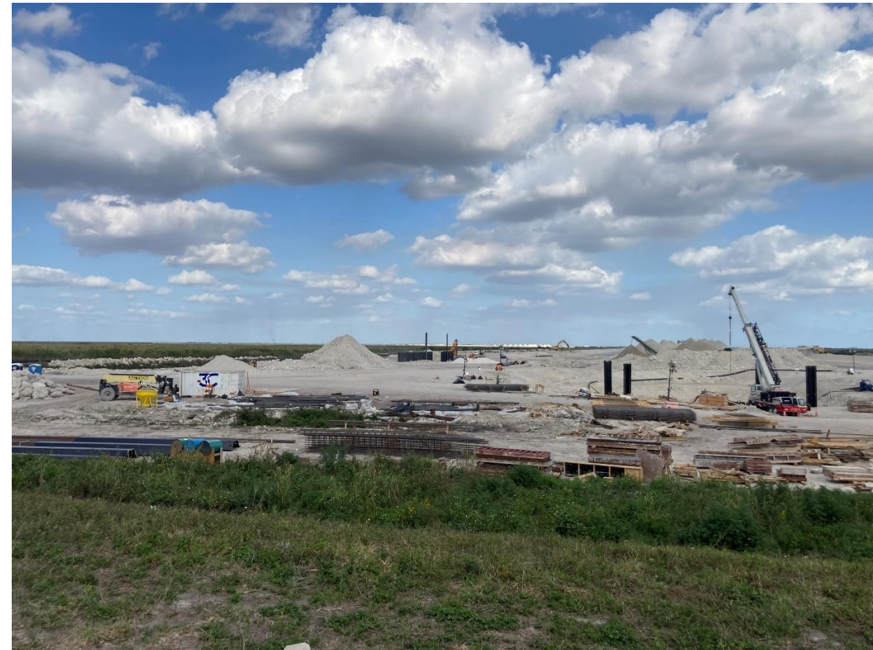
S647 Spillway Structure & S648 Seepage Pump Station
