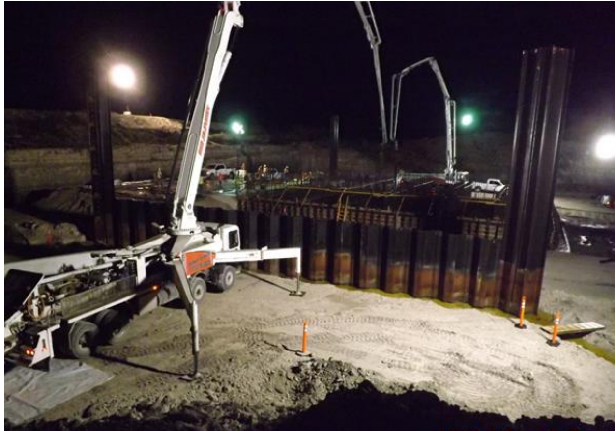
G-782 Base Slab Concrete Placement
