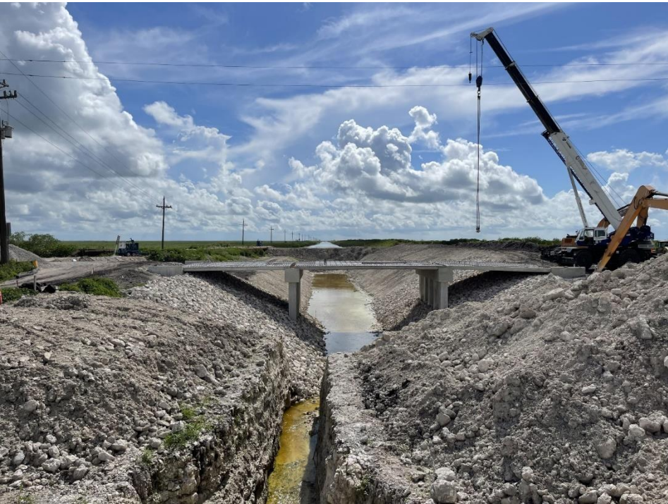
Slab Beam Installation
