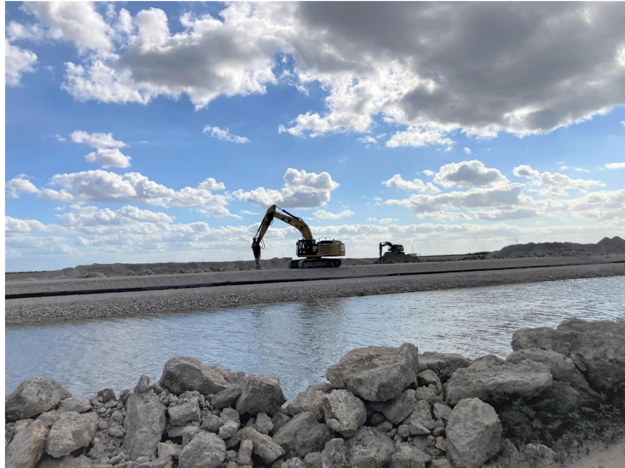
Inflow/Outflow Canal and Levee Construction
