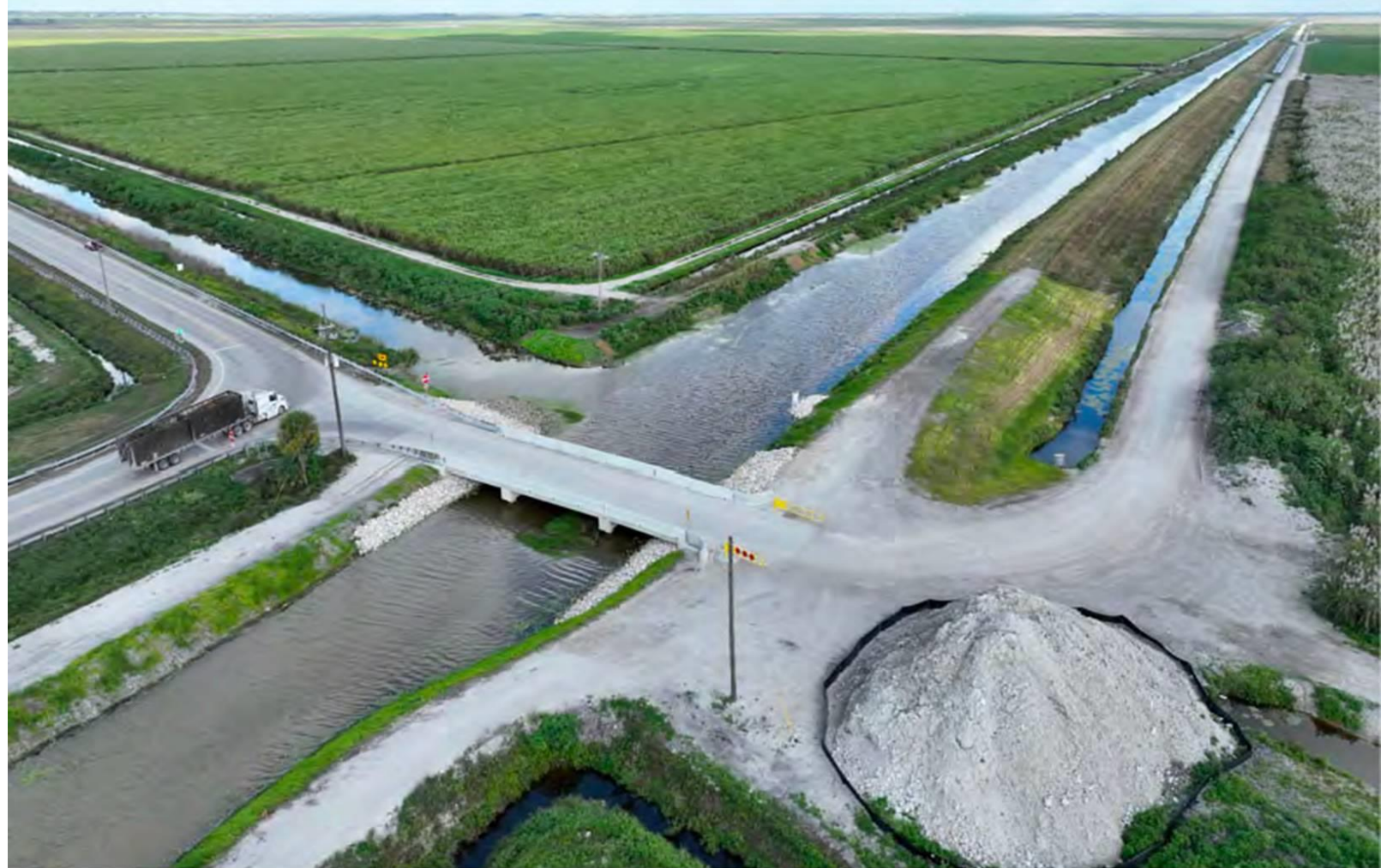
Completed Boca Chica Bridge and Canal
