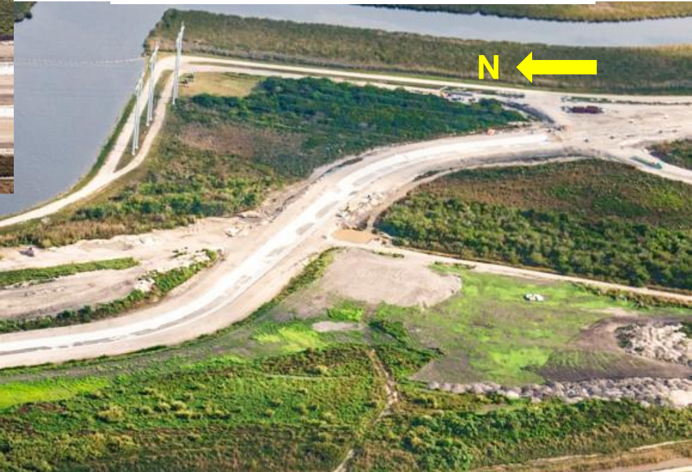
Northern Section of Concrete Conveyance Canal
