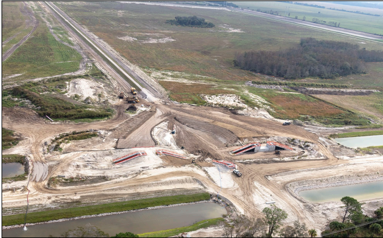
C-23/C-24 Stormwater Treatment Area, view S-432 Box Culvert Construction, December 2023
