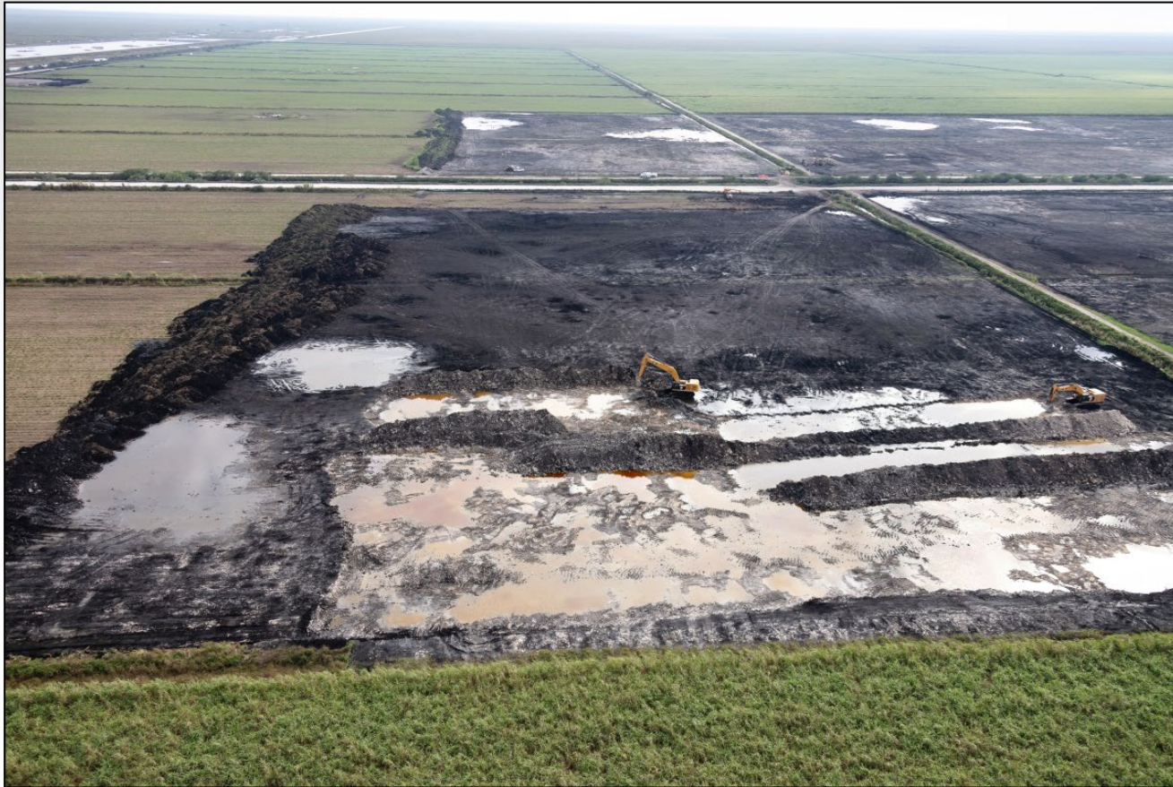
Everglades Agricultural Area (EAA) Reservoir - Foundation Preparation and Cutoff Wall, December 2023
