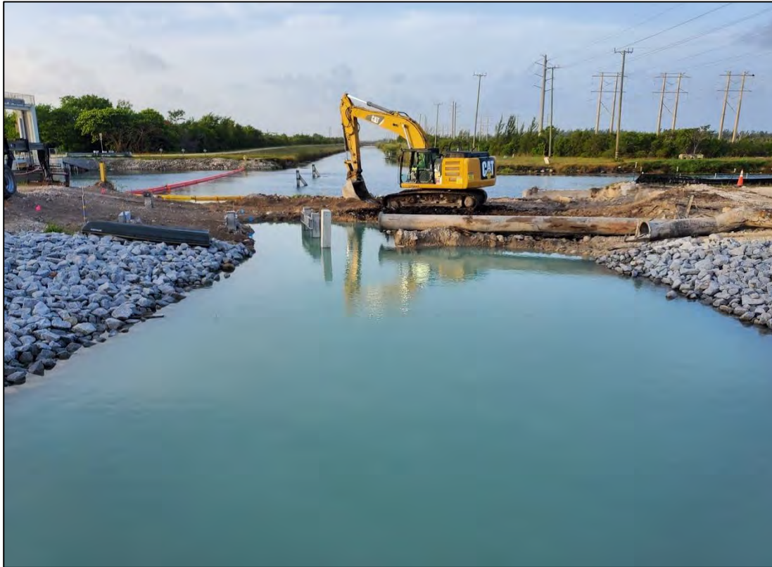
S-705 Construction Site
