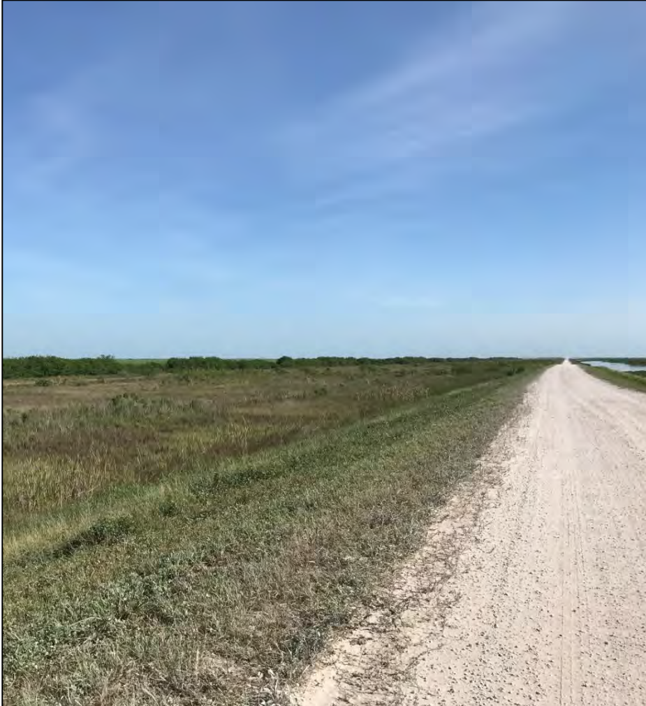
Everglades Agricultural Area Reservoir Site
