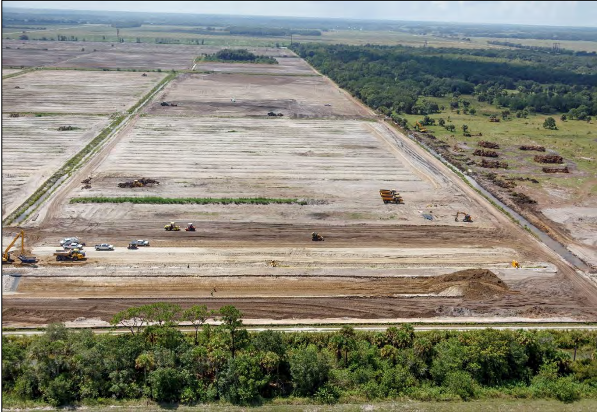
C-23/C-24 Stormwater Treatment Area Construction
