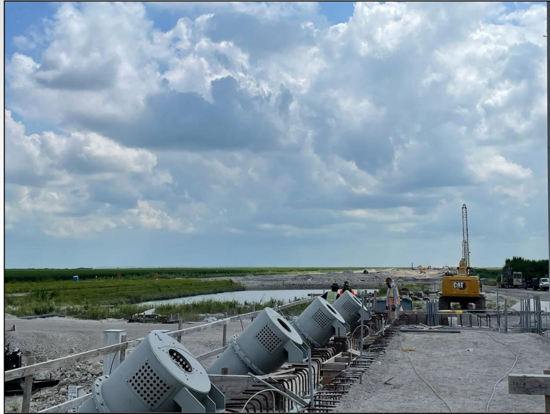
Everglades Agricultural Area (EAA) Reservoir, Seepage Inflow/Outflow Canal, August 2023
