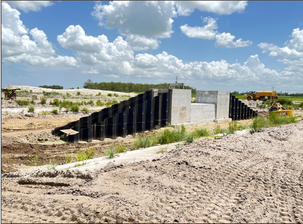
C-23/C-24 Stormwater Treatment Area S-432 Box Culvert Construction, Aug 2023
