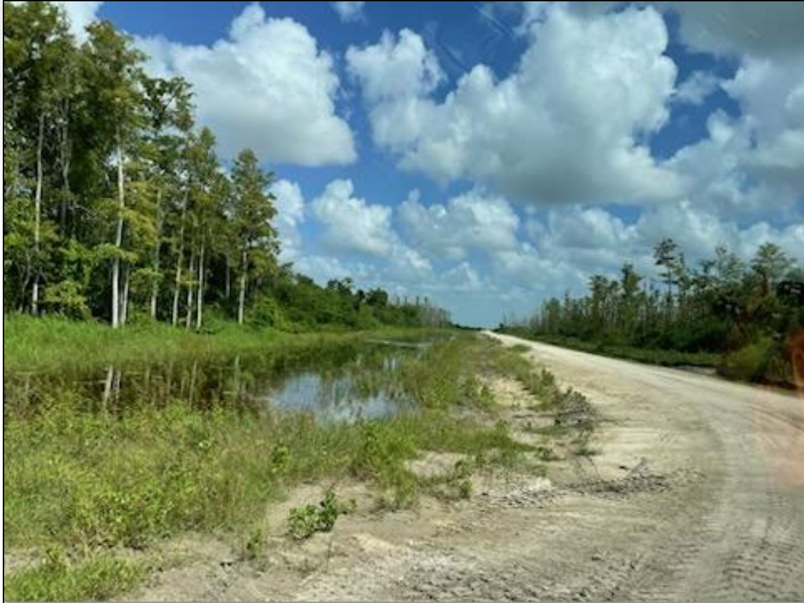
Levee Construction – Southwest Protection Feature Aug 2023
