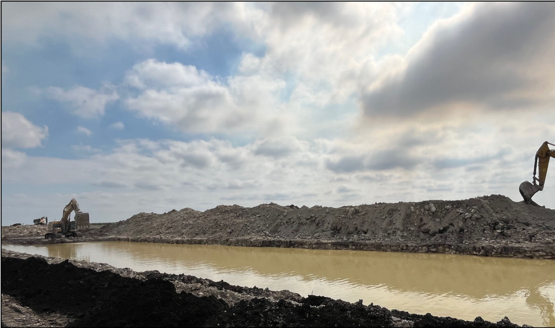
Everglades Agricultural Area (EAA) Reservoir - Foundation Preparation and Cutoff Wall, February 2024
