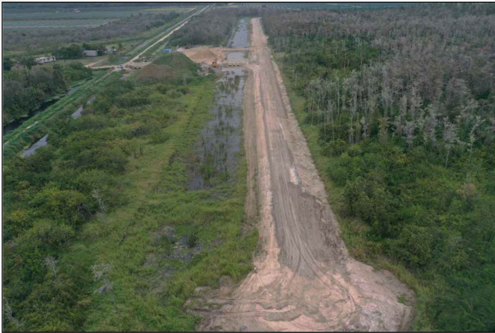
Levee Construction – Southwest Protection Feature December 2023
