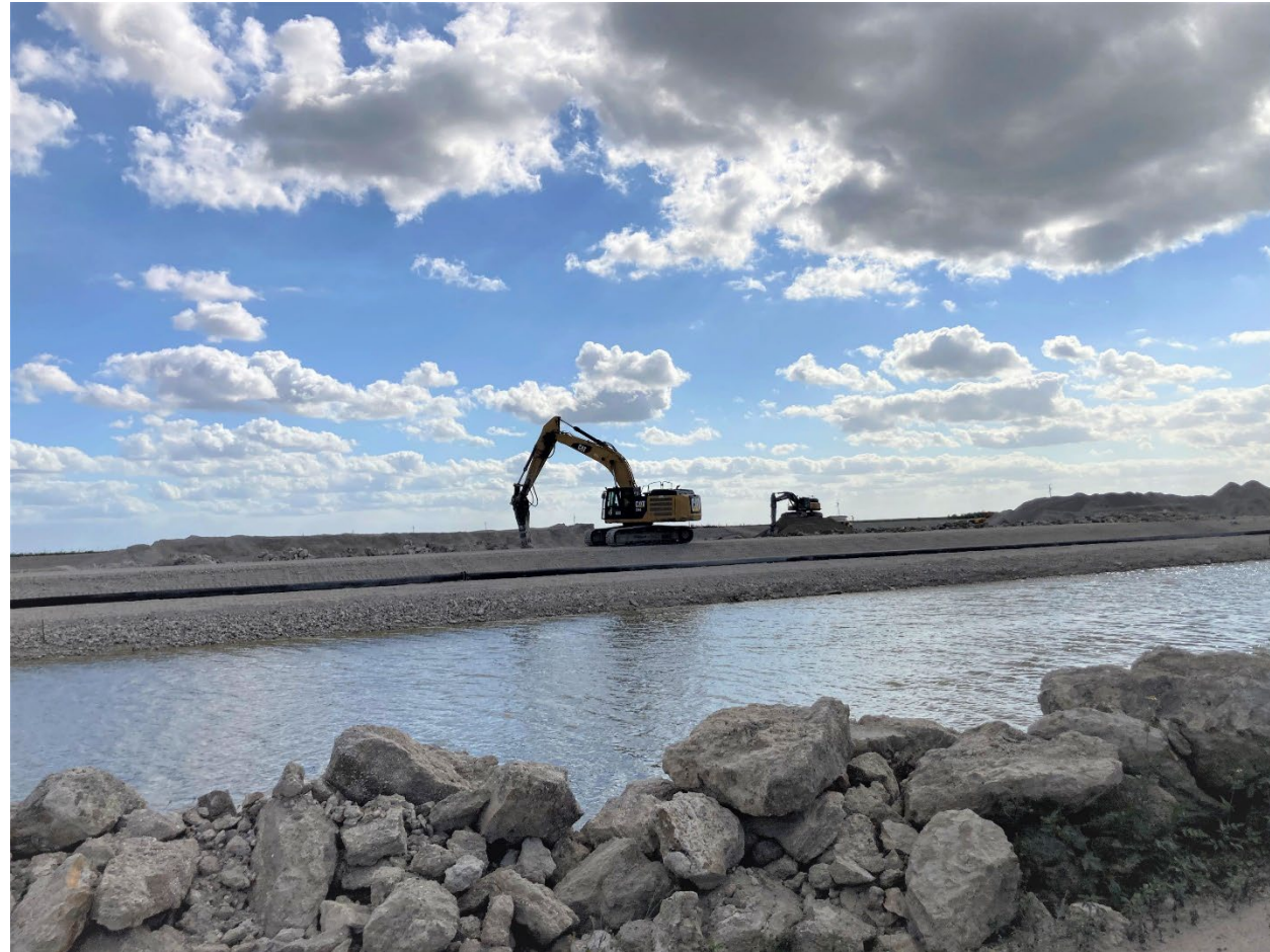
Inflow/Outflow Canal and Levee Construction
