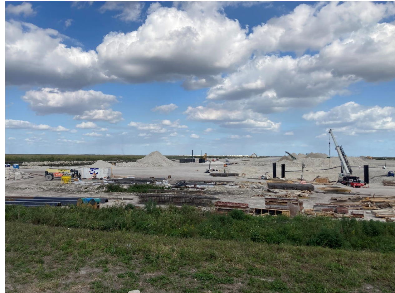
S647 Spillway Structure & S648 Seepage Pump Station
