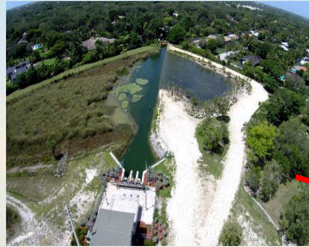
Deering Estate Pump Station (S-700)
