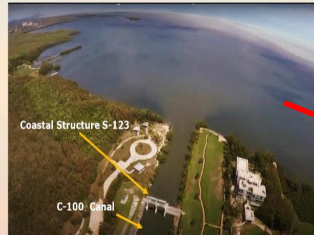
Coastal Structure S-123 on C-100 canal
