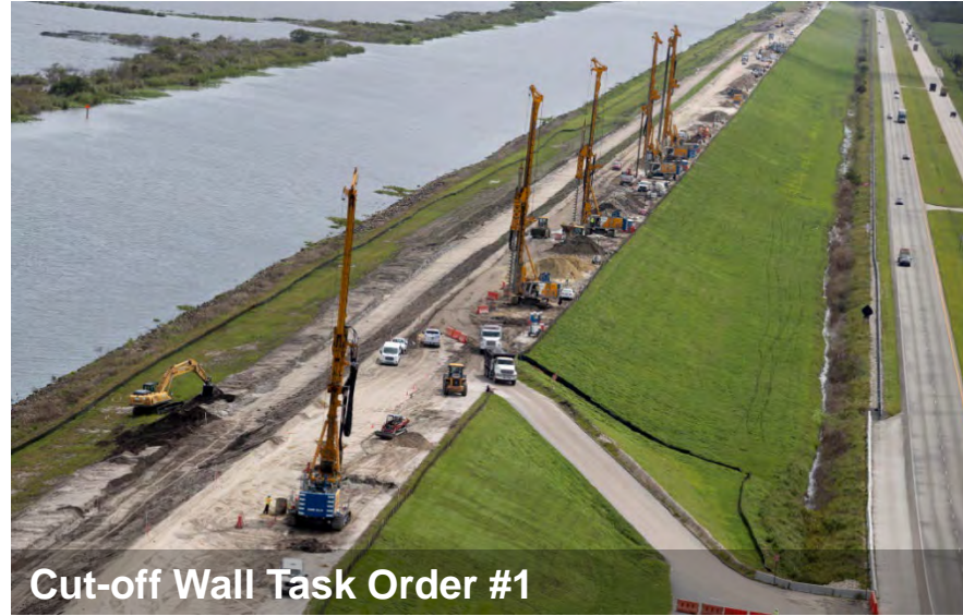
Reach 1 Cut-off Wall Extension
