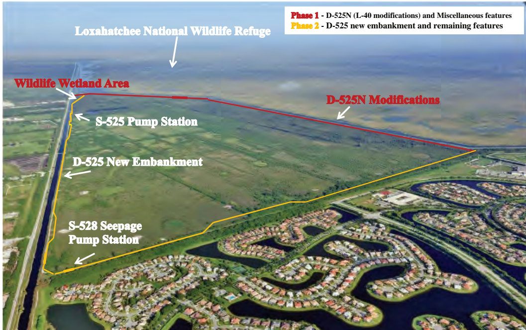
FIGURE 3-9 Location of the Site 1 Impoundment project, looking west-northwest. The Arthur R. Marshall Loxahatchee National Wildlife Refuge is at the upper right of the image. As with many restoration projects, Site 1 has a sharp boundary between its restoration area and neighboring urban development.
