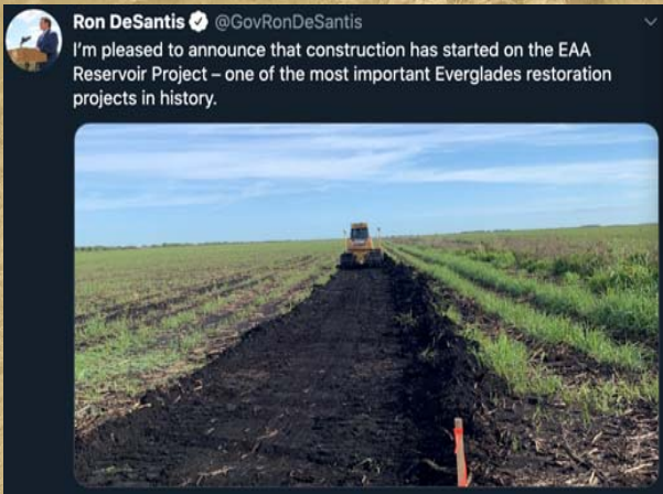
Broke Ground on EAA Reservoir Project STA
