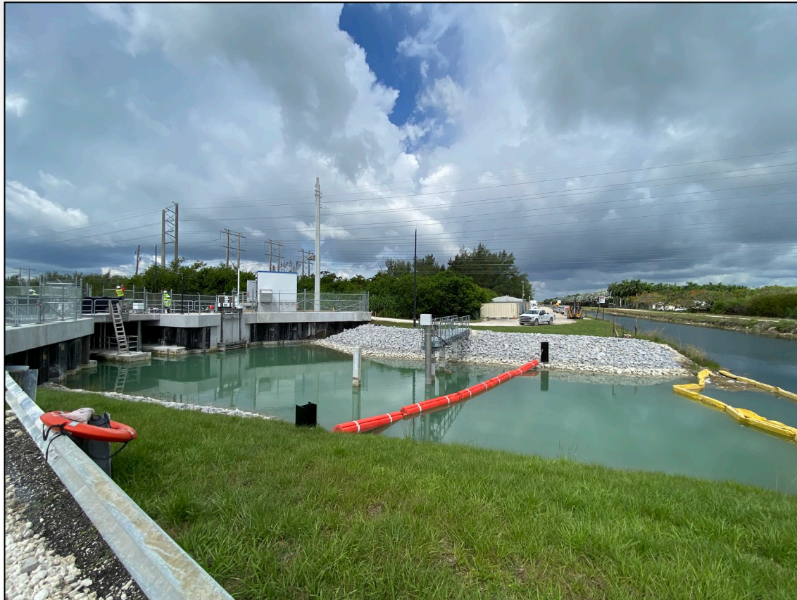
S-705 Construction Site
