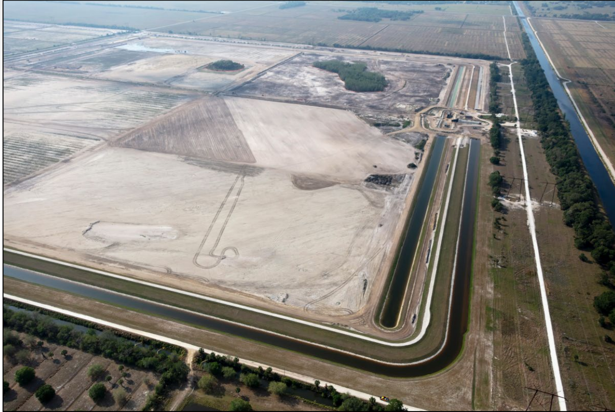
C-23/C-24 Stormwater Treatment Area Construction, April 2023
