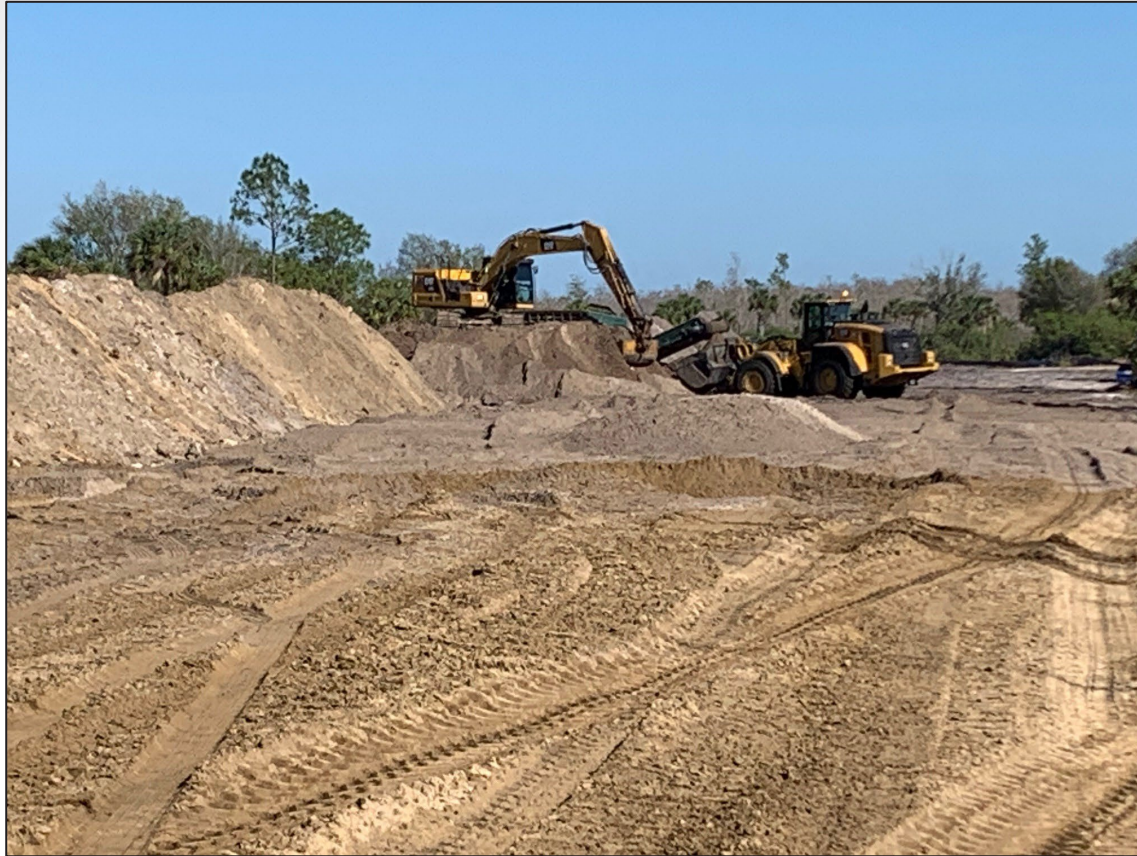
Levee Construction – Southwest Protection Feature May 2023
