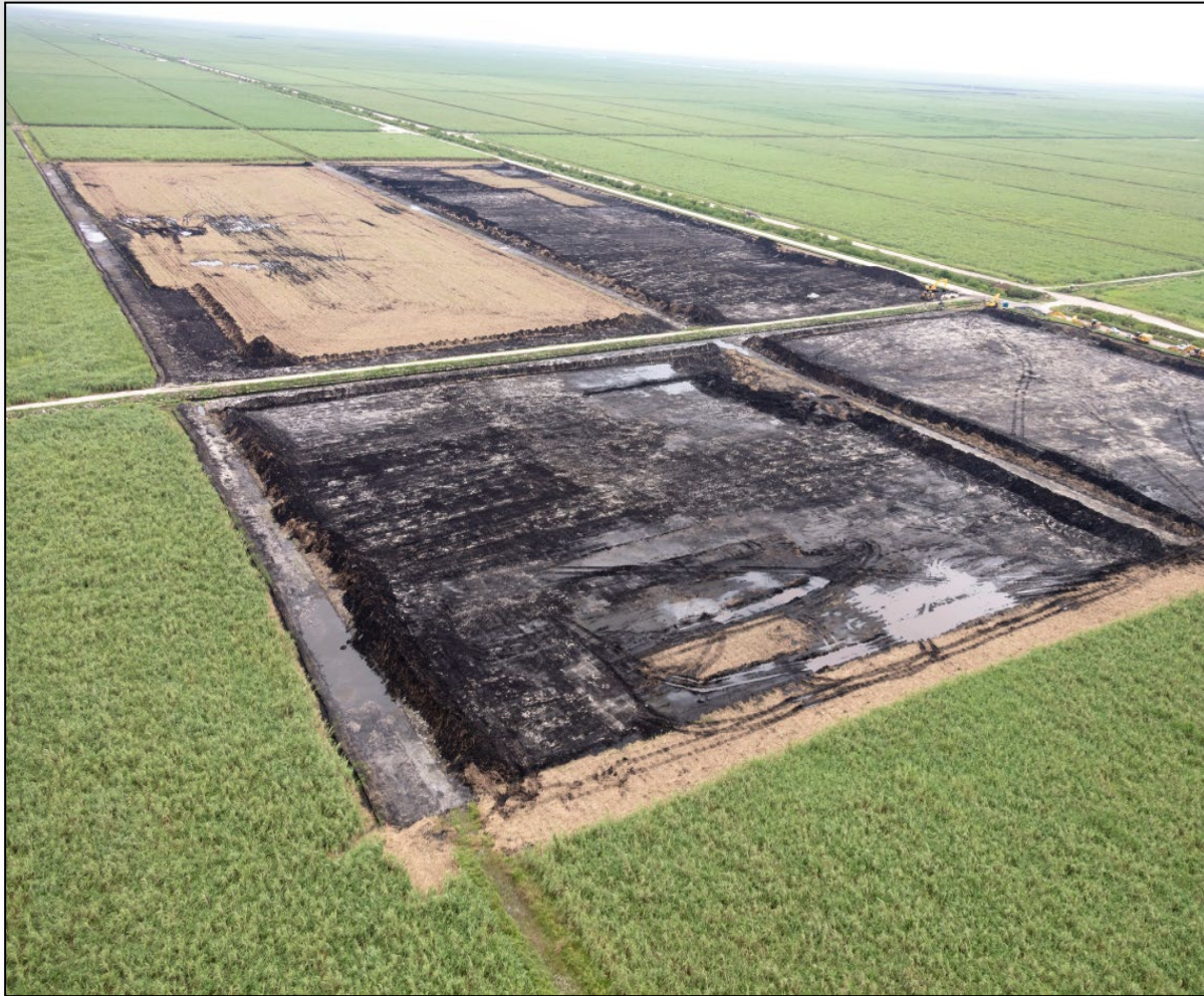
Everglades Agricultural Area (EAA) Reservoir - Foundation Preparation and Cutoff Wall, October 2023
