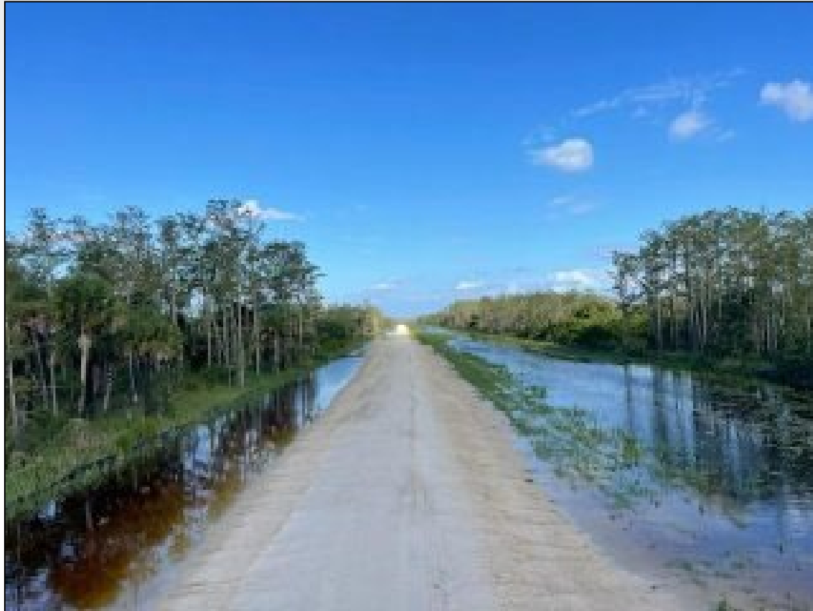
Levee Construction – Southwest Protection Feature October 2023
