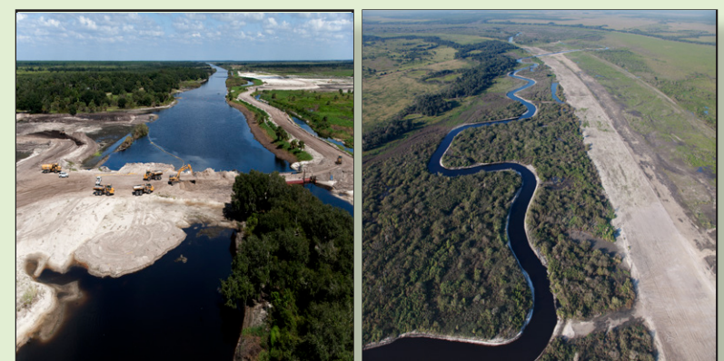
The Kissimmee River Restoration project will restore the channelized river back to its natural meandering flow pattern. This will provide natural floodplain storage and slow down the flow of water from the Kissimmee Basin into Lake Okeechobee, thereby slowing down the rise in the lake that often results in high-volume discharges to the Caloosahatchee and St. Lucie estuaries.
