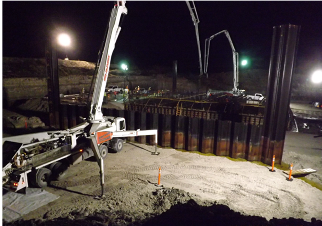
G-782 Base Slab Concrete Placement
