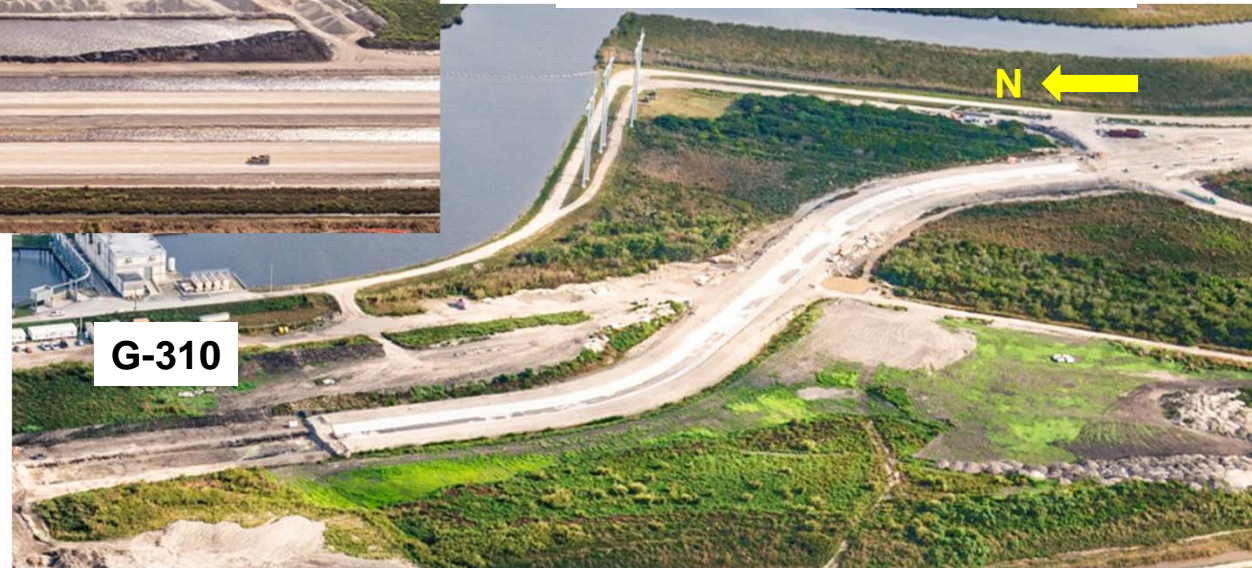
Northern Section of Concrete Conveyance Canal
