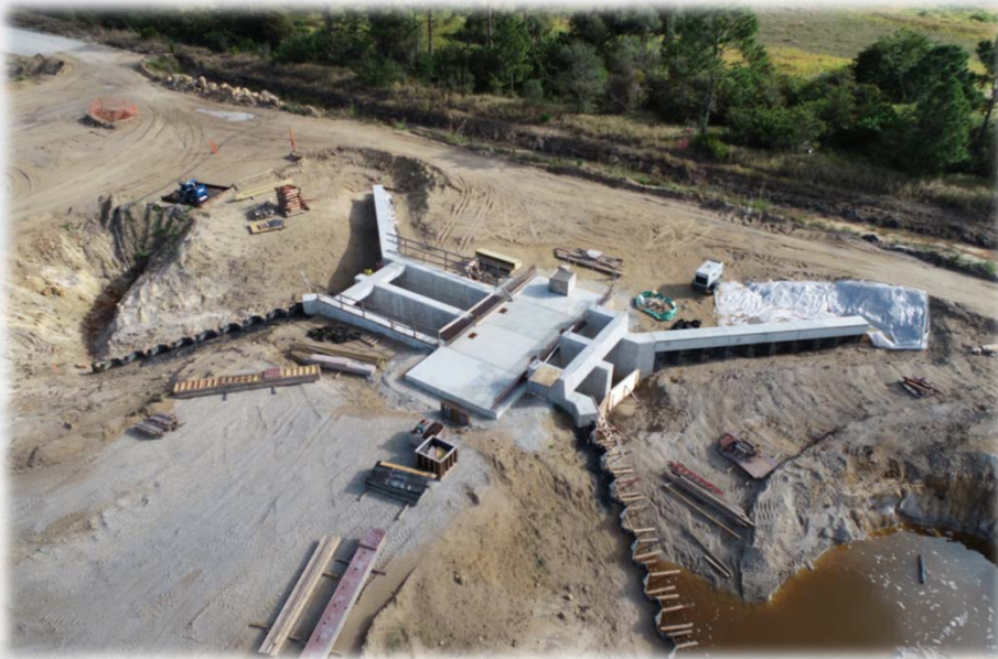
S-477 Western Perimeter Canal Structure
