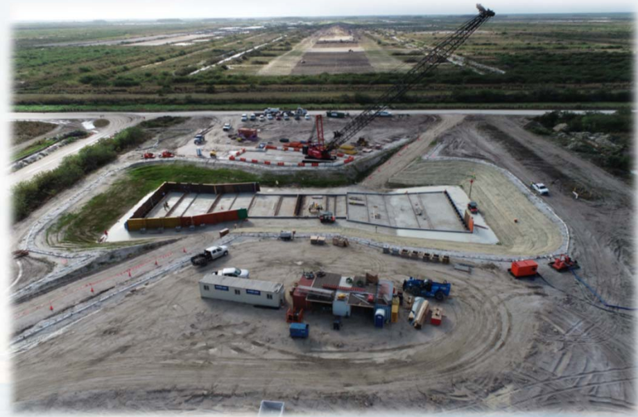
S-475 Cell Divide Structure
