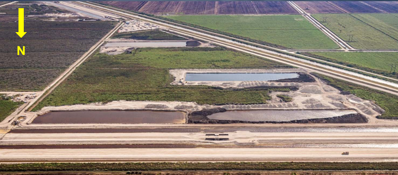
North Inflow Canal and Levee
