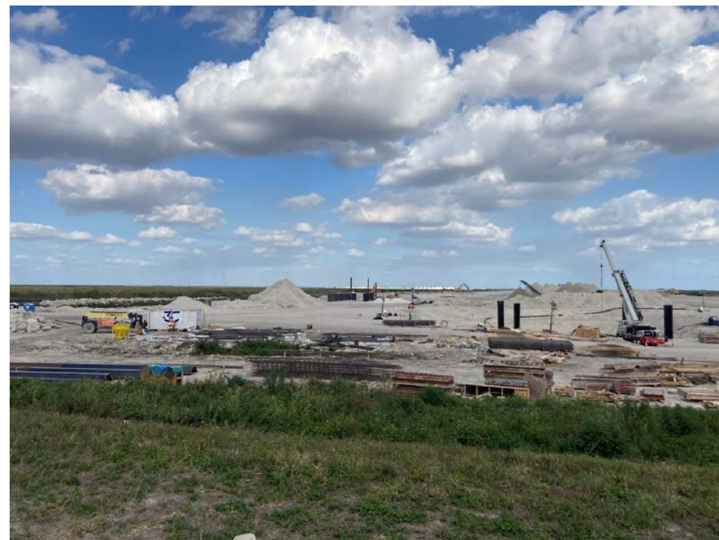
S647 Spillway Structure & S648 Seepage Pump Station
