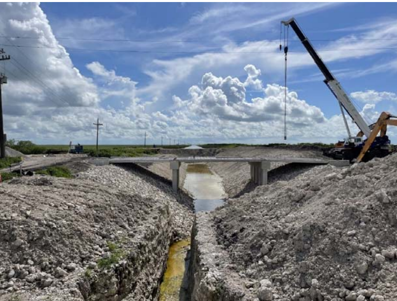
Slab Beam Installation
