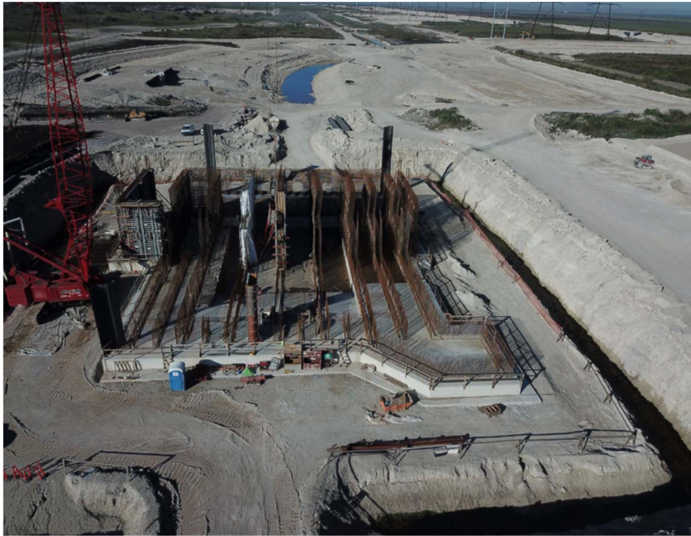
G-781 Building Pier Walls for Intake Bays
