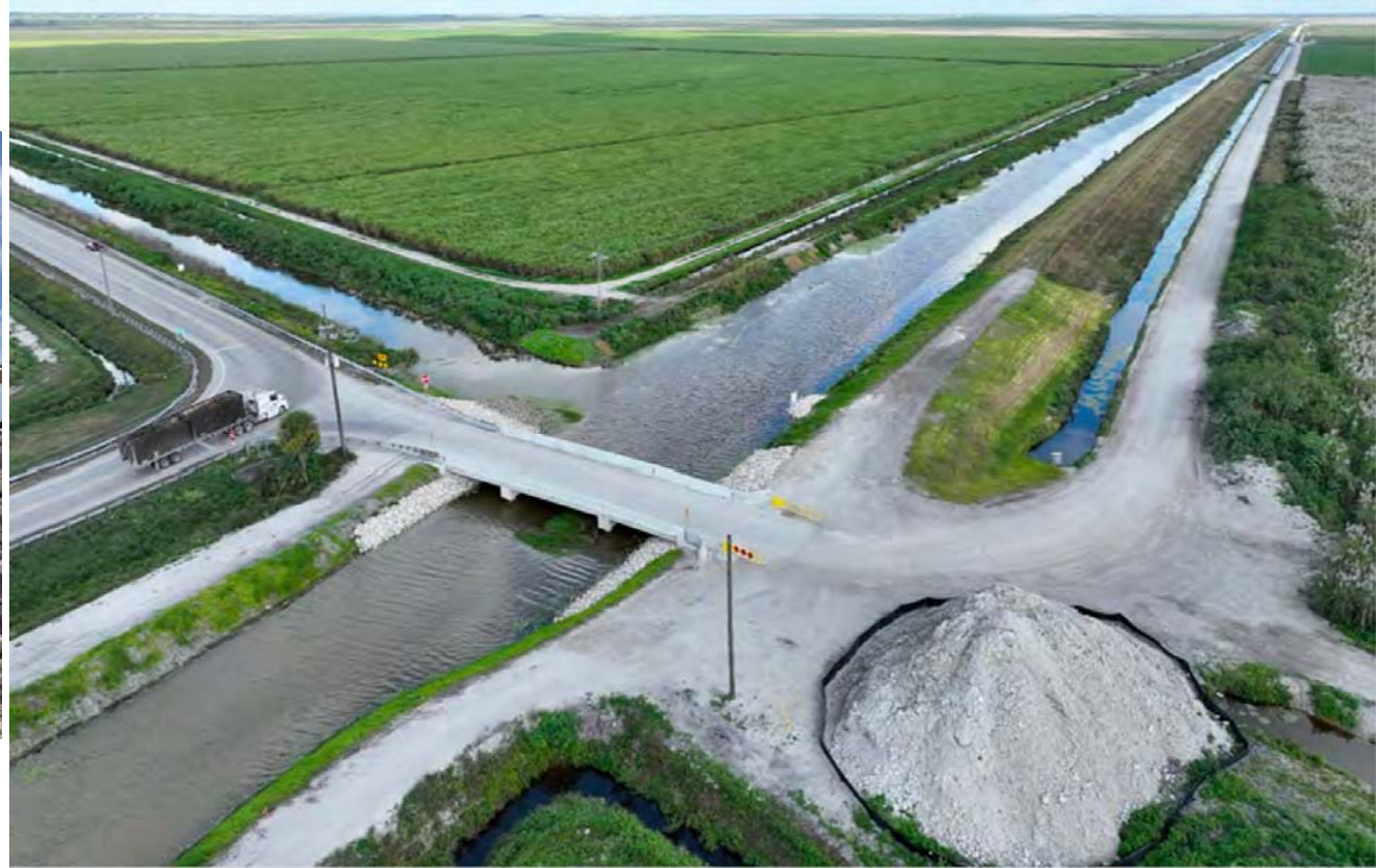
Completed Boca Chica Bridge and Canal
