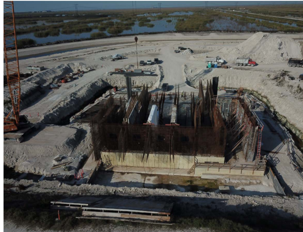
G-780 Building Pier Walls for Intake Bays
