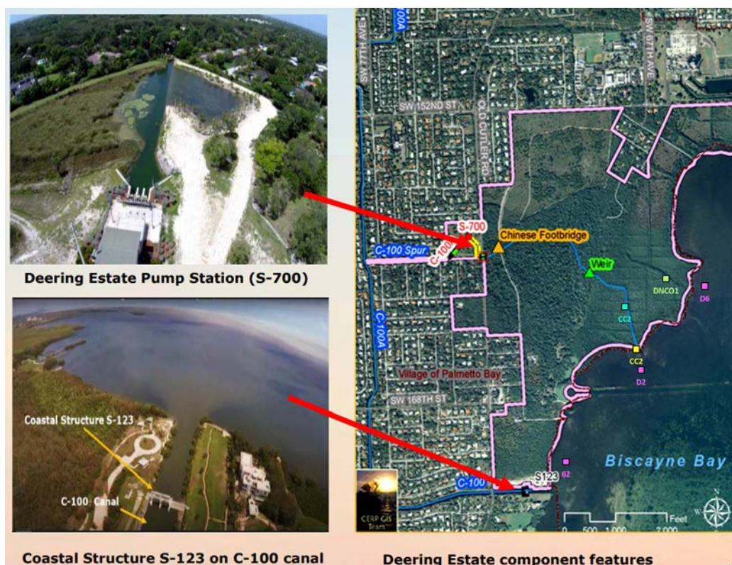
FIGURE 3-35 Deering Estate Component features, showing insets of the S-700 pump station, which diverts water from discharge in the C-100A Canal through the S-123 Canal structure. Purple colored squares are the project-specific salinity monitoring stations. SOURCE: Modified from Charkhian, 2022a.
