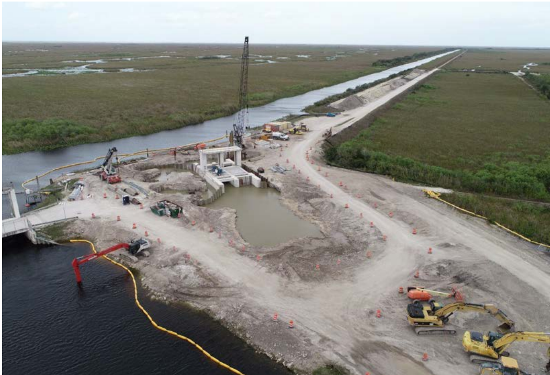
Figure 1-6. CEPP South, Structure S-333N Construction in Water Conservation Areas. Photo: SFWMD.
